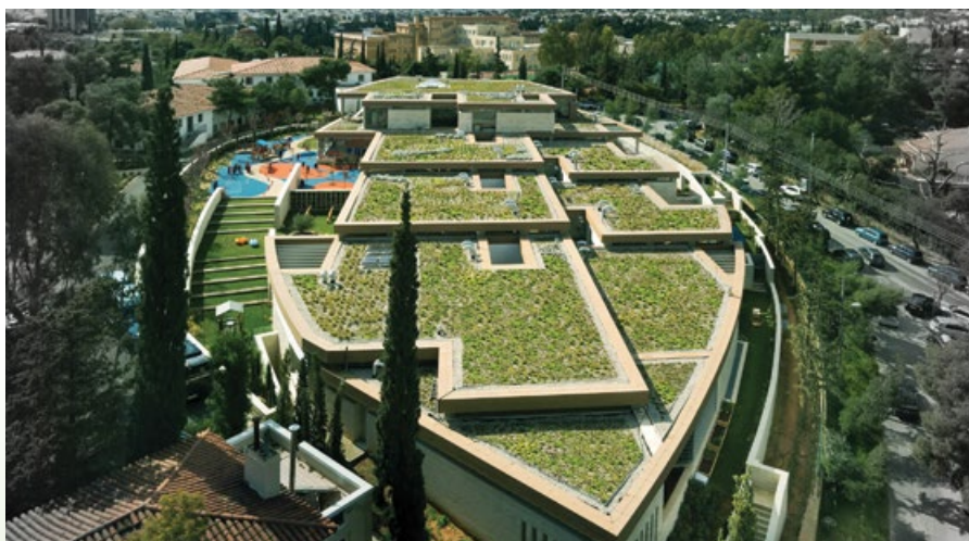
The Hellenic American Educational Foundation (HAEF) preschool & kindergarten is an educational facility certified with LEED v3 Schools in 2014. It is the only educational building in Greece with "green" certification
